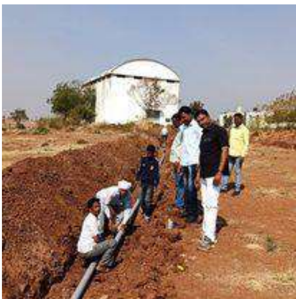
Excavating canal to Ley pipeline
